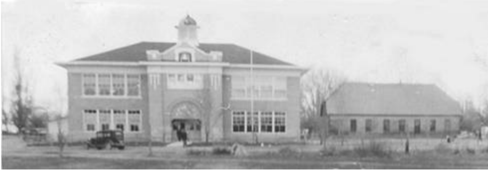
Cleveland Elementary School and the Davis Opera House built in 1912
